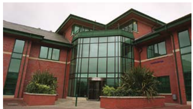
Zen's primary data backup facility at TelecityGroup, Manchester.
